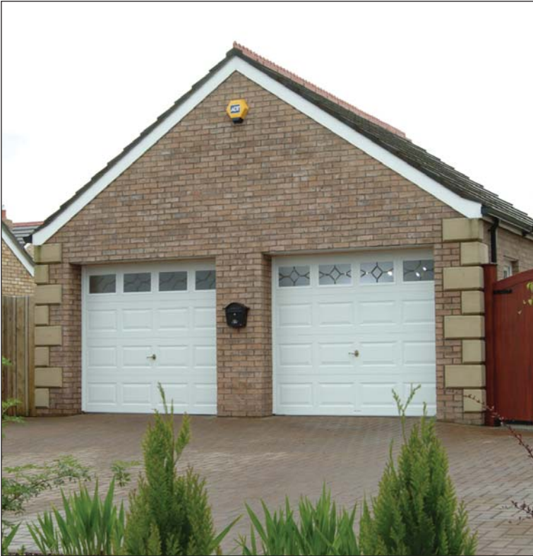
Single Weatherguard Doors with Chalet windows.
