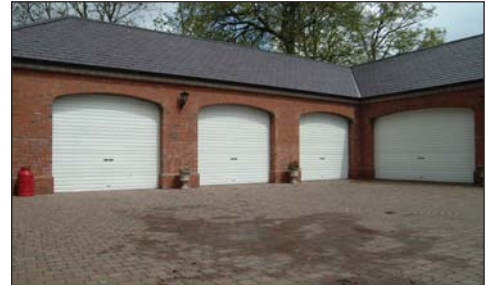
Roller Doors in arched openings.
