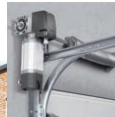
Teckentrup Direct Drive motors must have 16 amp supply direct to the consumer unit.
