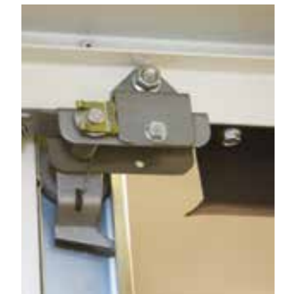
Anti drop mechanism. Large spindle roller. Spindle roller bracket has a reinforcement bracket to stop excessive movement.
