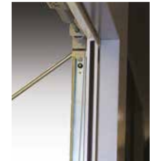
Anti drop mechanism. Large spindle roller. Spindle roller bracket has a reinforcement bracket to stop excessive movement.
