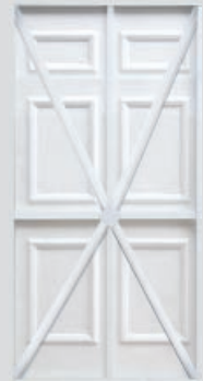
The neat inner face and steel bracings
