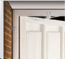
White stays hold the door in the open position preventing slam closure in windy conditions
