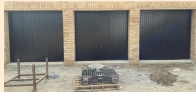
Garage doors installed by us on the Bellway site at Stanton Cross, Wellingborough. The "Garador Carlton"
